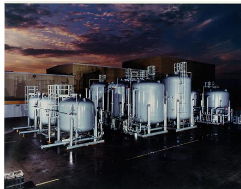
Figure 4: Tanks at the Manufacturing Plant.
